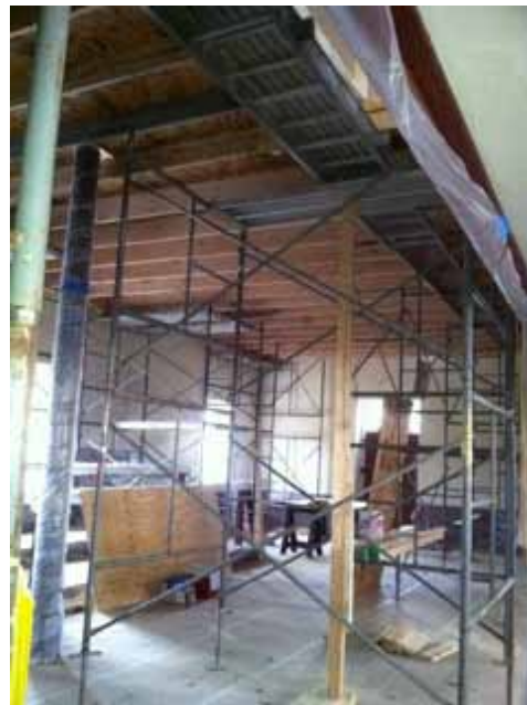
Hopewell's ceiling gets new plaster
